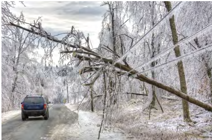
Ice storm impacts power lines
