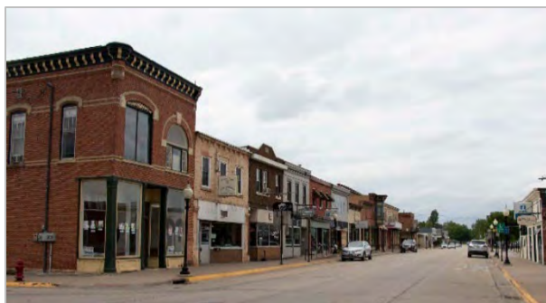
Bellevue Commercial Historic District Source: 2022 NRHP Nomination
