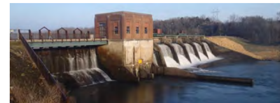
Maquoketa hydroelectric power plant. Photo Credit: http://renewableworldenergies.com
